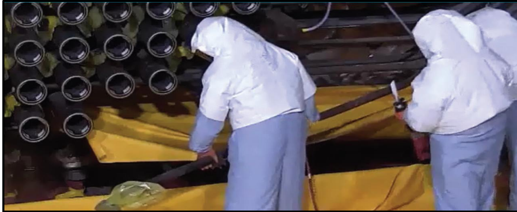
Unit 2 Feeder Removal at the Darlington site.
